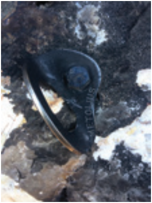
RIGHT On Silverado Squatters, old 3/8” bolt was successfully removed and a new 1/2” x 5” bolt placed. It’s a lot more work to re-use the same hole, but worth the effort when possible.
